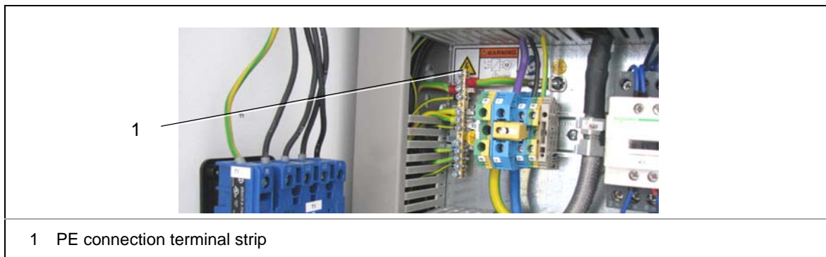
Figure 66: Protective - equipotential bonding conductor connection
