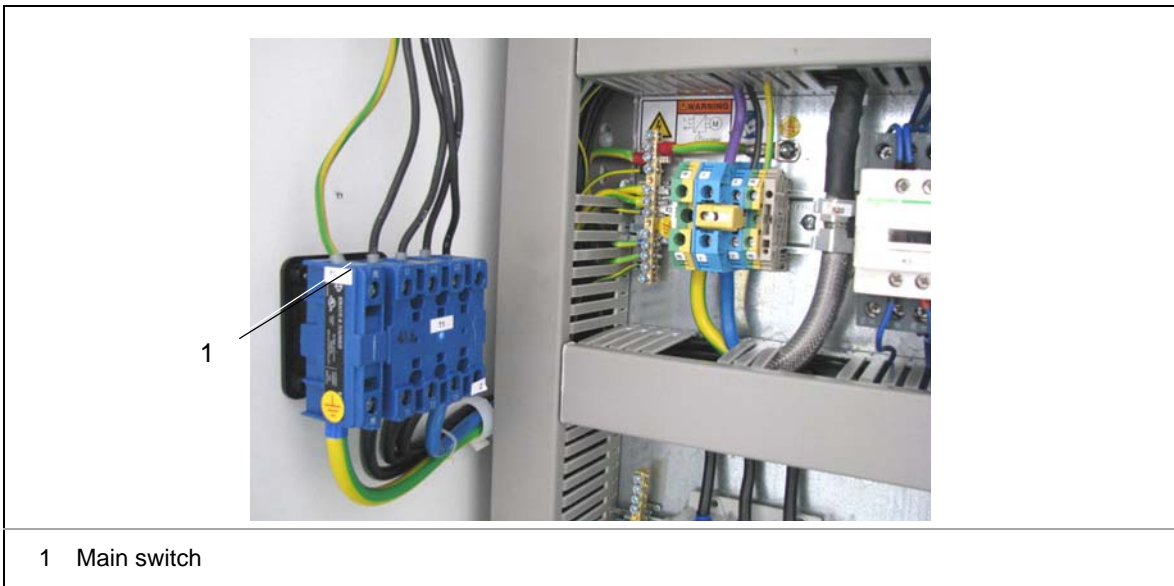
Figure 65: Stationary mains connection
